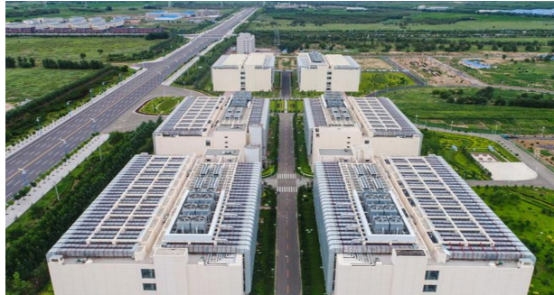
Fig. 1-1. World's biggest data center as of 2023, China Telecom Data Center Inner Mongolia Information Park [1].
